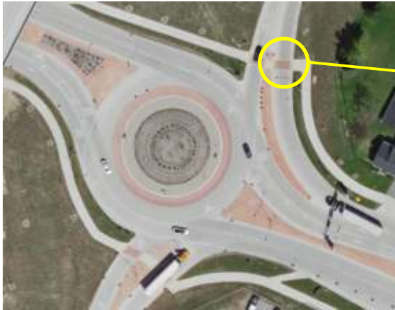
Figure 2 - 2014 Aerial Imagery (Pre 2016 Sealing)
