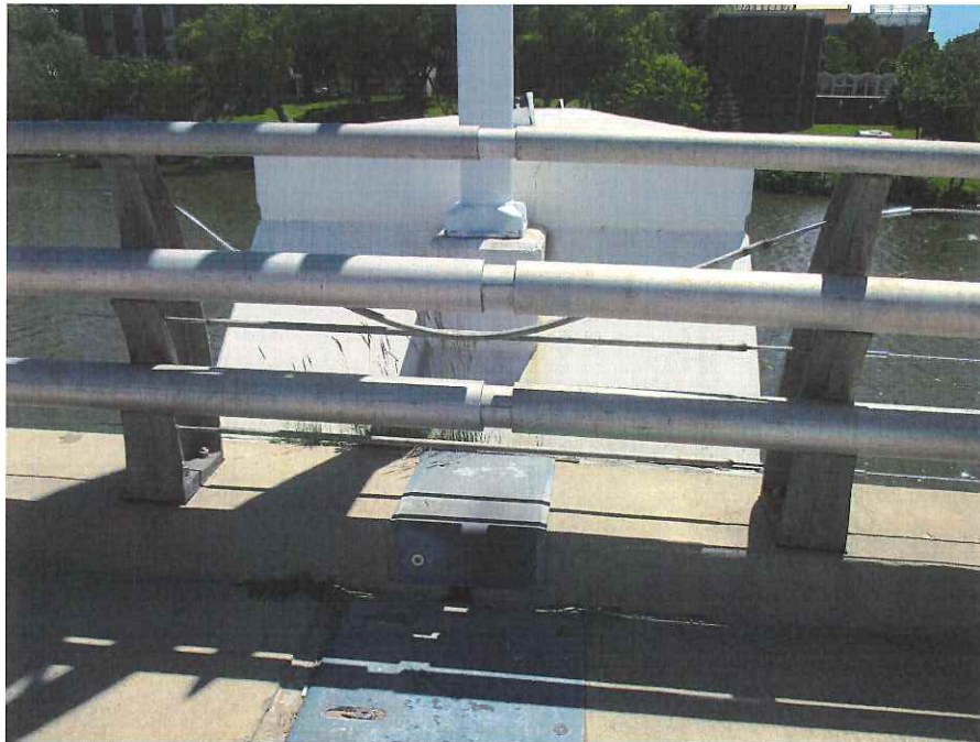
Figure 2. South Side, third pier from West bent cable
