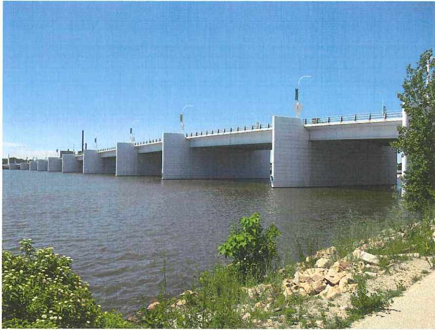
Figure 1. Claude Allouez Bridge as seen from the Southeast side
