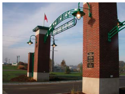
Arch Columns w/Lights
